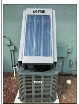
There are two (2) total systems in the house. There is a 3-ton system that provides heating and air conditioning to the 2nd floor. The 2-ton solar system is providing the cooling for the main floor of the house.
